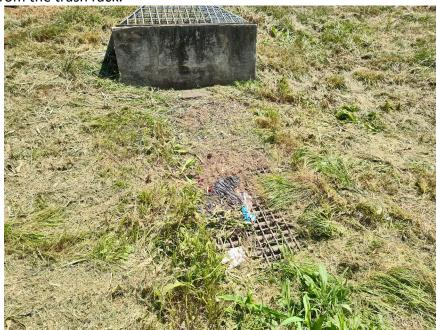
Inlet pipe with outfall concrete channel showed signs of separation which resulted in erosion around structure in 2018. University staff replaced the structure to prevent further erosion on outfall channel. New structure remains in good shape and no signs of erosion.
