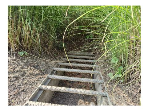
Add riprap to the outfall section. Noted sediment of gravel mixture buildup at outfall. Source was traced to parking lot. Monitor and remove sediment and debris as needed.
