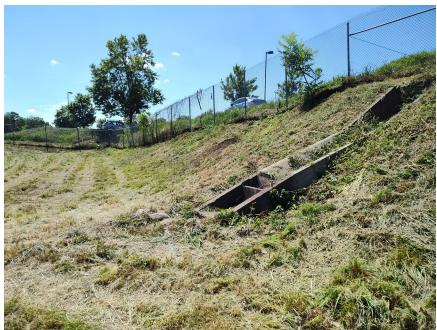
Nuisance animals had been noted to be in the area of the BMP and have been caught in recent years. RU staff to keep traps out and fill holes immediately. Recent inspection discovered additional signs of holes along the downstream portion of the basin. Set traps to capture vermin and remove from the area. Recommend increasing the schedule for mowing to allow for better inspection of the berm structure.
