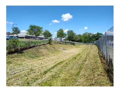
Sediment from the parking lot and road area above consists of small gravel deposits. Those deposits have collected in the center of the pond bottom. This has caused the upper section of the pond to not fully drain to the riser section. It is recommended to remove the sediment/gravel deposit form the center of the pond and reseed. This will help drain the pond faster after a rain event.
