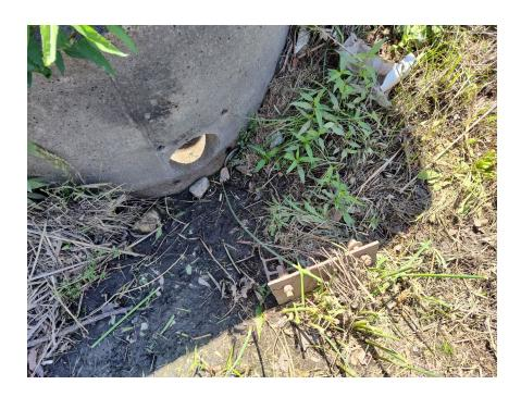
As reported in the last inspection, the berm area near the gas line installation shall continue to be monitored for seepage or compromise. No signs of erosion or seepage during this inspection. It is recommended to address the berm section by adding fill to the area. Slopes may be adjusted internally to keep the same volume for the pond to ensure that storage remains adequate. Over time this has the potential to fail for a higher storm event.
