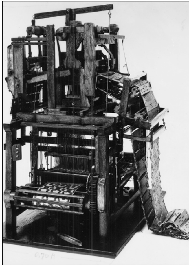
Figure 1-1, The Jacquard loom, using a string of punched cards that feed into the machine
