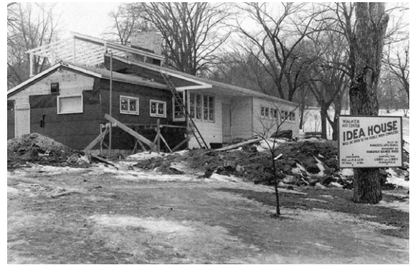
Fig 3. Idea House I under construction, 1941, Malcolm and Miriam Lein, architects
